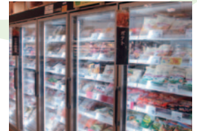
Refrigerator showcase using natural refrigerant (CO 2 ) installed at Aeon Makuhashi New City Store
