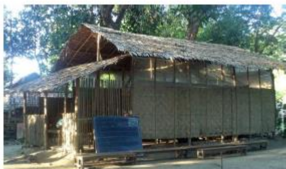
School building in Myanmar with a straw-thatched roof
