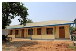
New school building in Myanmar
