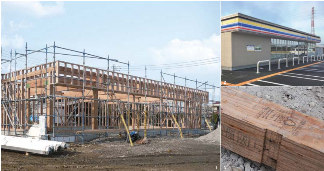
1. Ministop wooden framework completion 主体结构完工的Ministop 2. Completed wooden store (Ministop Fukaya Omaeda Store) 竣工的木结构店铺 (Ministop深谷小前田店) 3. FSC-certified timber waiting to be reused 可再利用的FSC认证木材
