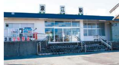
Namie Station of JR Joban Line. The section between Namie and Tomioka Stations will reopen in March 2020, giving easier access to Tokyo.
