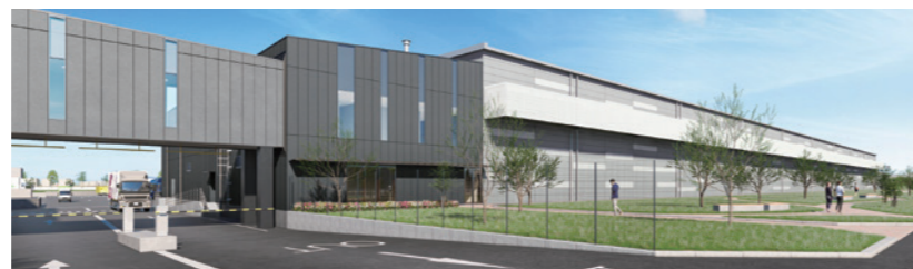
Image of the first CFC (Customer Fulfillment Center) scheduled to start operation in 2023
