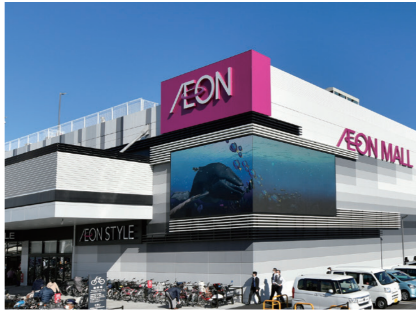
Aeon Mall Ageo using 100% renewable energy opened in Dec. 2020. Aeon has set a target to shift the electricity used at all 150 Aeon Malls in Japan to 100% renewable energy by 2025.
