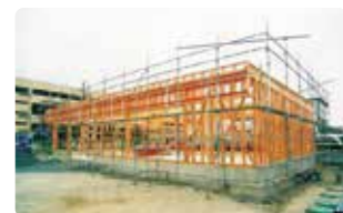
A Ministop store under construction
