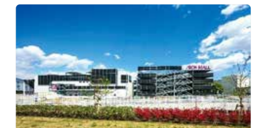
Solar wall (Aeon Mall Zama)
