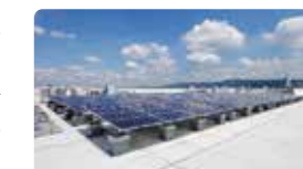
Solar panel installation
