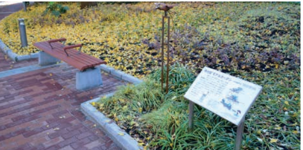
Rain Garden™ Rainwater contaminated with substances found in exhaust gas risks disrupting ecosystems. Rain Garden™ reduces the negative impact on the ecosystem by allowing rainwater to penetrate the ground, purifying it.
