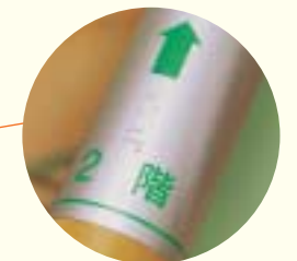
Braille plates for guidance are placed on stairway handrails.
