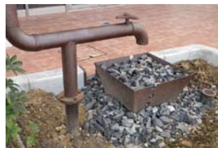
The Rain Garden™ project to filter rain water through top soil instead of transmitting it directly to sewage pipes
