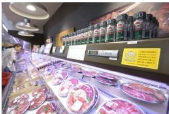
Refrigerator showcase using natural refrigerant (CO 2 ) installed at Maxvalu Shin-funabashi Store
