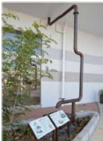
[At Rain Gardens, the rain water is collected and seeped into the soil for the use by the garden plants.]
