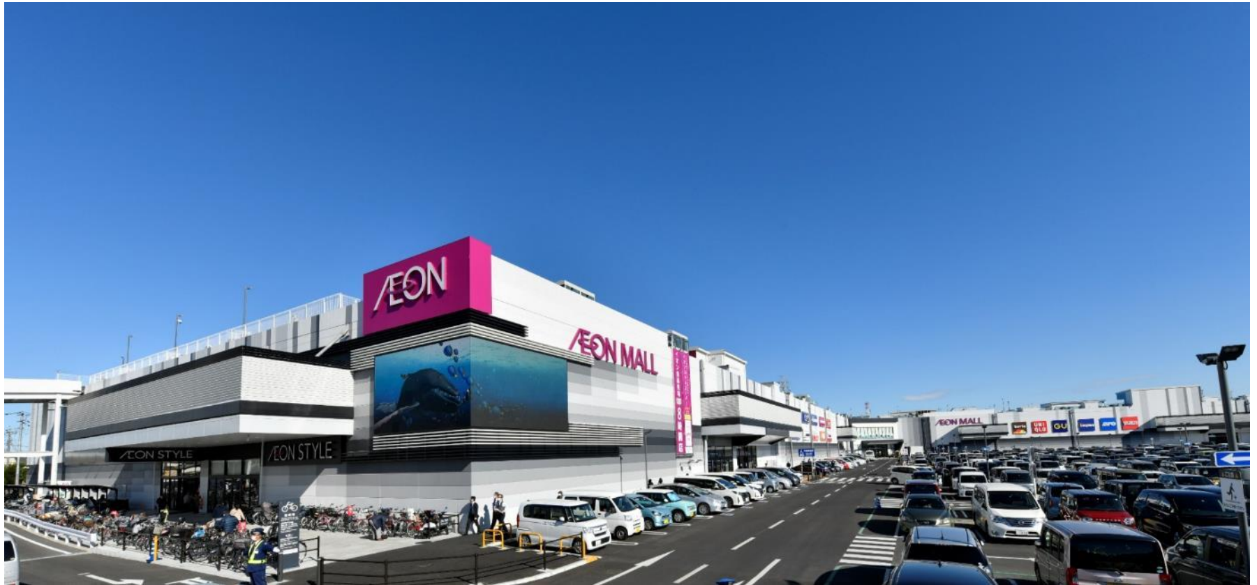
AEON Mall Ageo, which is operated with 100% renewable energy
