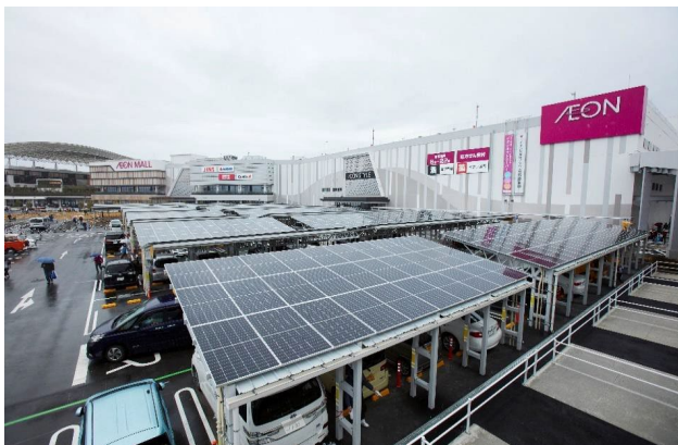
Solar Carport at AEON Mall Toyokawa (Aichi prefecture)
